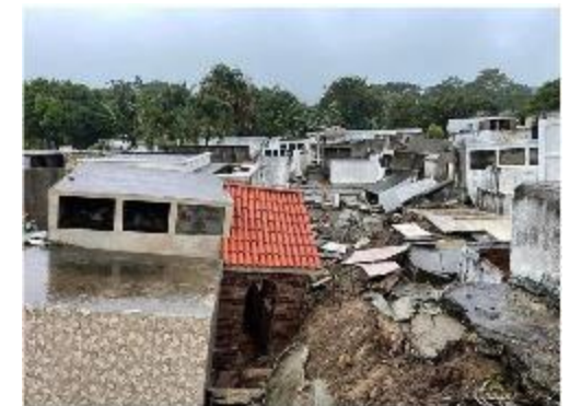
Photo: Structural damage to buildings, Colombia, November 2022. Photo: Government of America
